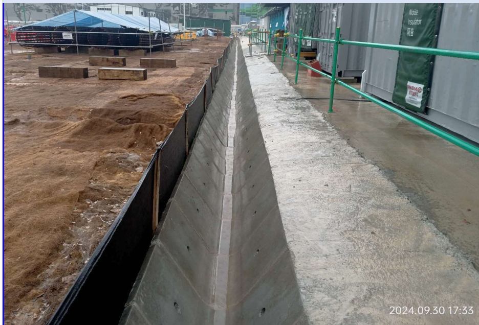
Perimeter Cut-off Drain With Silt Fence and Silt Trap Installed
