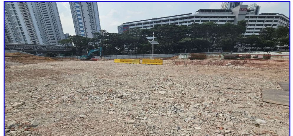
Laid Hardcore to Finalized Excavation Level Areas to Minimize Silty Runoff
