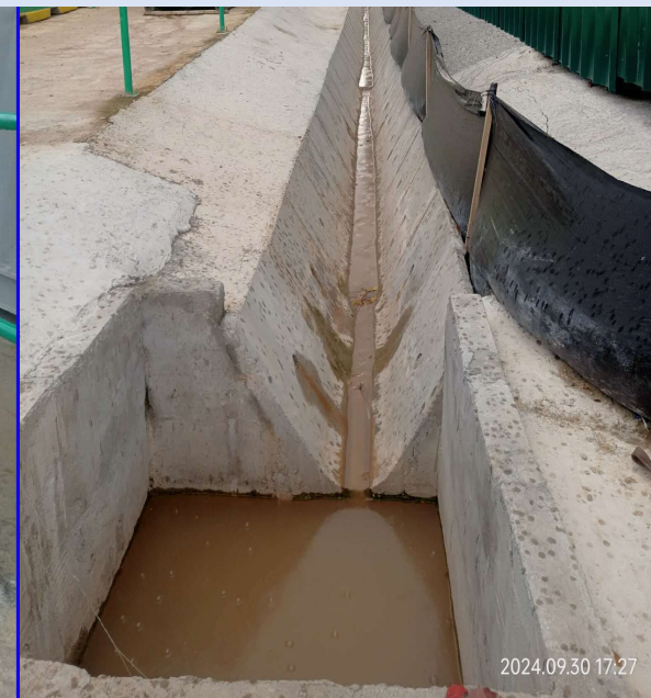
Perimeter Cut-off Drain With Silt Fence and Silt Trap Installed
