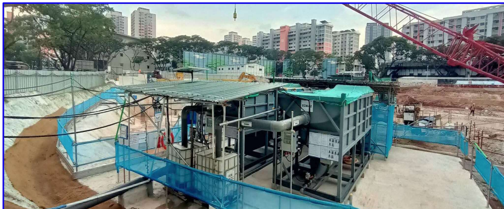
Setting up of ECM – Treatment Plant
