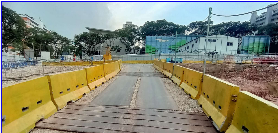
Laid Hardcore to Access Paths Under Steel Plate to Minimize Silty Runoff
