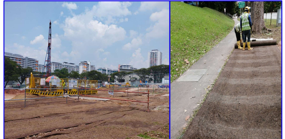
Exposed Areas Near to Public Area's/Walkways Covered With Fire Retardant Type ECB
