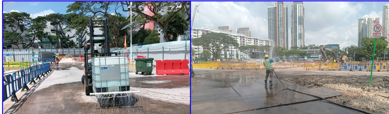
Dust Control Spraying
