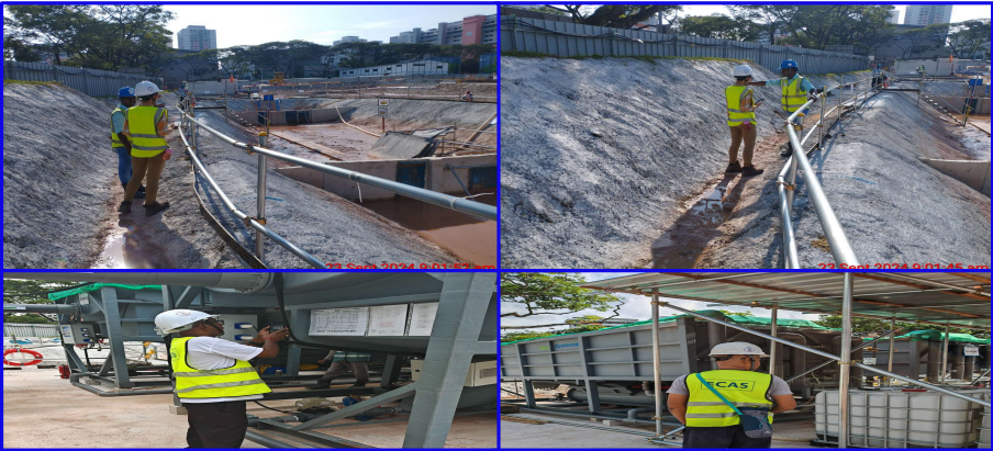
Weekly Joint ECM Inspection by QPS and ECMO
