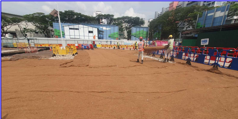
Exposed Areas Covered With ECB
